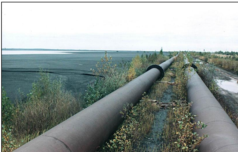
Photo 1. Hydraulic mine dumps near the Mikhailovka Mining and Processing Plant. Water is supplied through pipes to flood the waste rock. Otherwise aeolian processes can lead to contamination of the territory. After a while, water birds can settle in these wetlands (phot. by A. A. Chernyshev)
