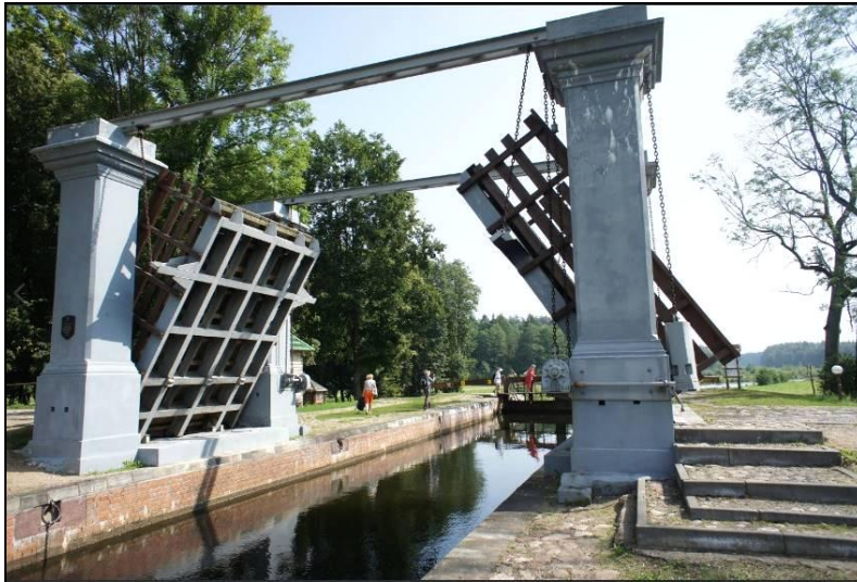
Photo 3. Moveable bridge in the front of Dombrovka shiplock (phot. by A. V. Sobisevich, 2013)
