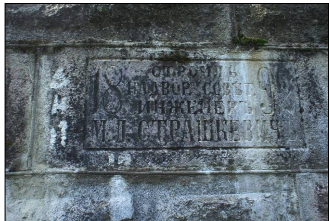
Photo 1. A stone block on the canal wall with the name of its engineer (phot. by A. V. Sobisevich, 2013)
