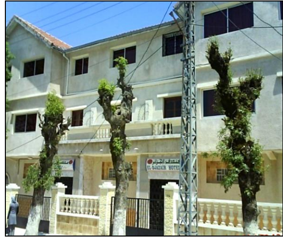
Photo 9 – Fot. 9 – Φοτ. 9: El Djazair hotel (source: field survey)
